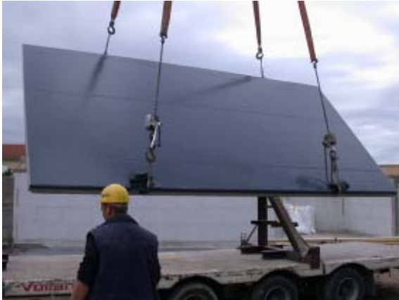
Abb. 6: Oberschale an Montageankern
